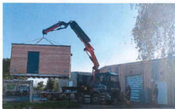
FIGURE 29 MODULE COMPORTANT LA CHAUFFERIE GRANULES
